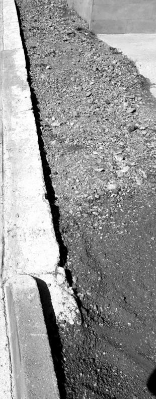
2. Filling the sidewalks joining the sidewalk with a sand-cement mixture.
